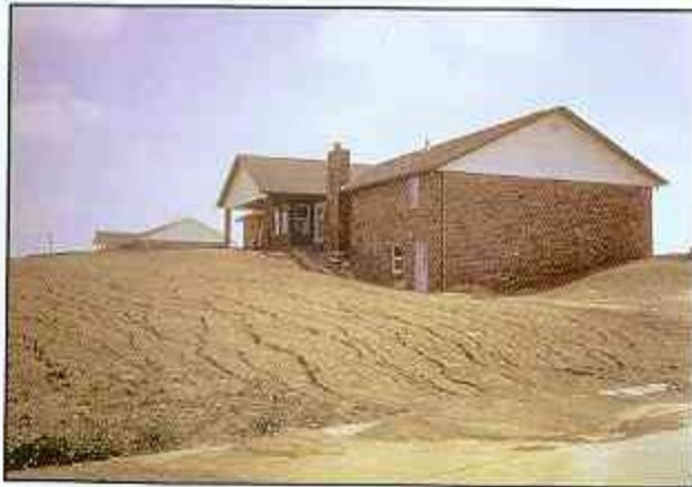
Uncontrolled erosion degrades water quality and costs time and money to repair.
