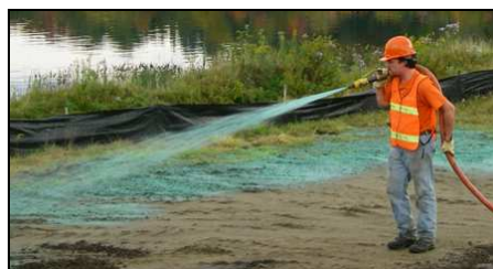
Hydroseeding the Lake Abanakee Causeway.
